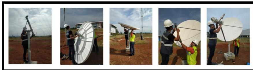
Gambar 4. Proses Instalasi Antena VSAT
